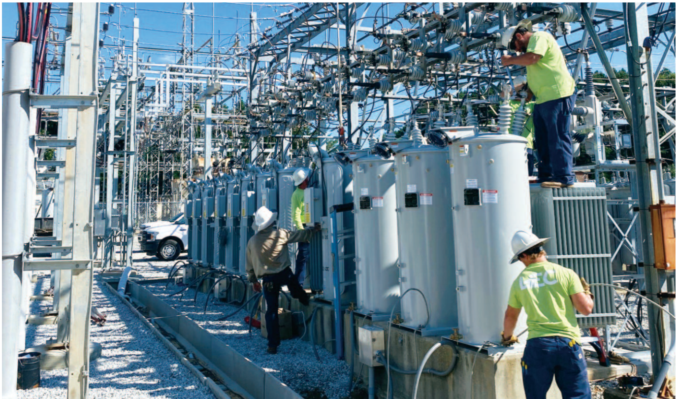
CREWS INSTALL REGULATORS AT SUBSTATIONS, WHICH KEEP VOLTAGE LEVELS WITHIN ACCEPTABLE RANGES AND MAINTAIN POWER QUALITY AND RELIABILITY.
